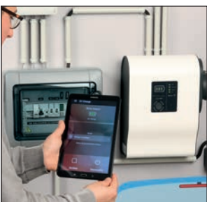
The charging station communicates via Wifi or Bluetooth. The locally created wifi network is specific to the model. It is isolated from the WiFi network of your establishment.
