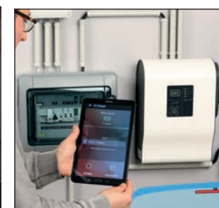
The charging station communicates via Wifi or Bluetooth. The locally created wifi network is specific to the model. It is isolated from the WiFi network of your establishment.
