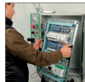
System for attaching and quickly removing the grid in the closet.
