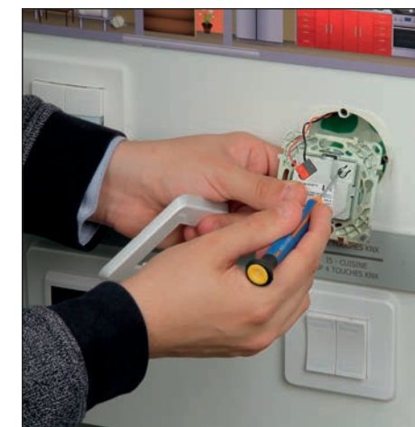
The set of switches of habitat type and KNX are integrated on the front panel. A translucent plate on the universal adapter, covers the connectors and protects electrical contacts, only the programming buttons remain accessible. The push buttons are very easily removable to facilitate access for programming.
