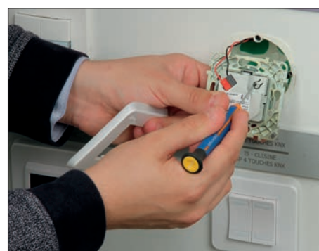
The set of switches of habitat type and KNX are integrated on the front panel.
